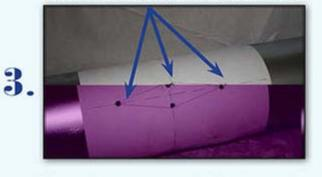
Place damper carefully into slot and drill out mounting holes
