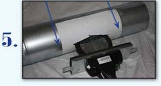
Attach template to Pipe/Duct with tape \*damper installs in the direction of the air flow\*
